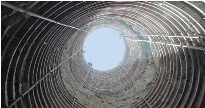
Rampur HE Project - Himachal Pradesh (432 Mw) Asia's largest Surge Shaft with 38m dia
